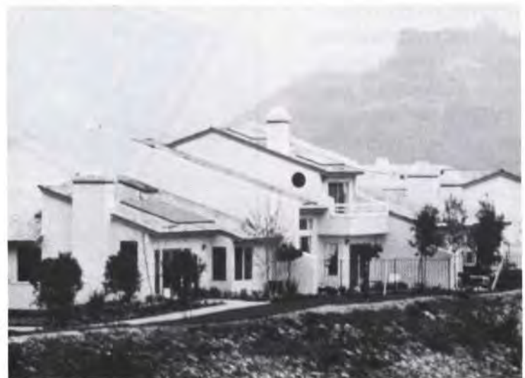
These Laguna Del Mar townhomes use PV to supply part of their electricity. They also use the local utility as a backup to store any extra power they may produce. An extra meter on each home monitors the electricity fed back to the utility company.
